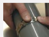
4. Hold down any excess band while finally tightening.
